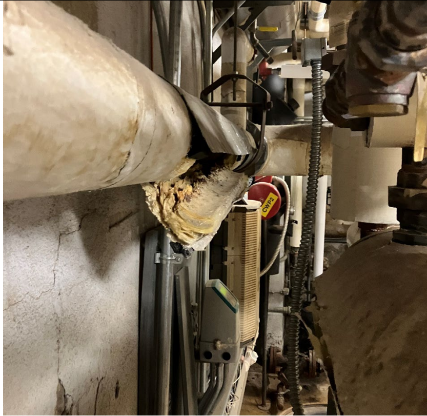
Mumford Hall – Room M31 – View of Fiberglass and Plaster on Wall – Plaster is Negative for Asbestos.
